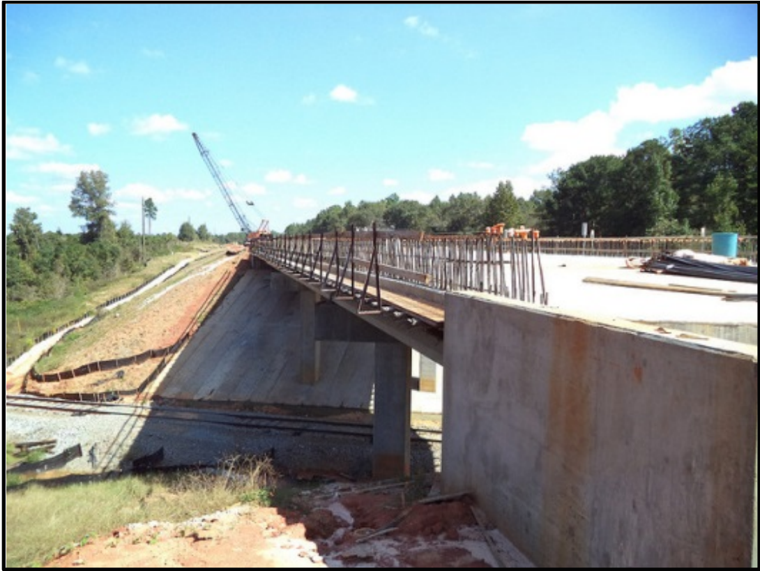
SR 1 US27 Bridge Replacement –Before Construction
