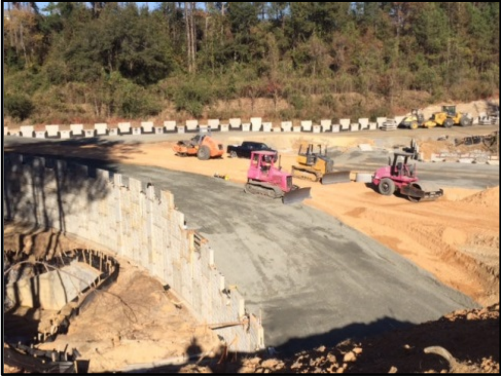
Muscogee County, Custer Road Interchange - In Progress
