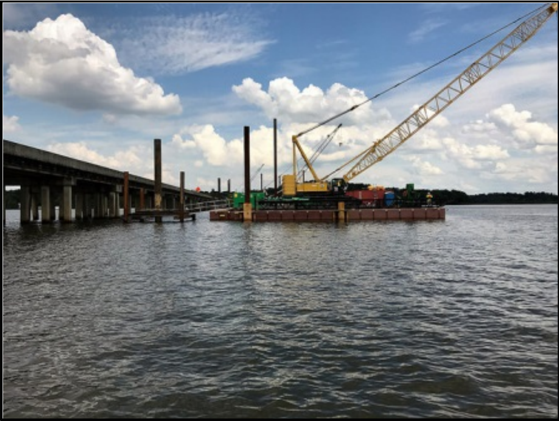
Crisp County US Highway 280 Bridge Reconstruction – Before Construction
